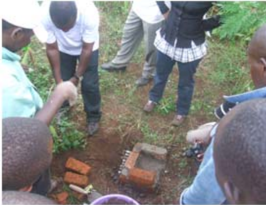
Establishment of runoff plots in Lwiro micro-catchment.
